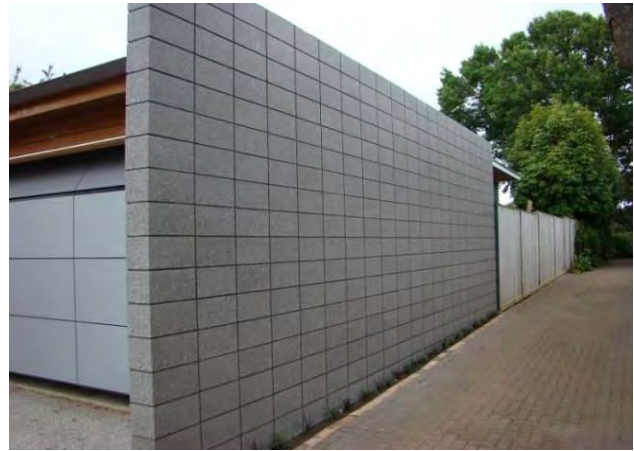
Figure 3: Coloured Honed Blockwork
