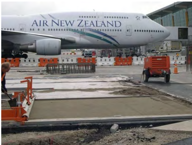
Figure 30: Christchurch Airport Apron Slab 80 mm Pavers
