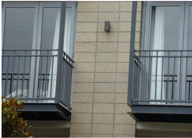
Figure 2: Coloured Honed Blockwork
