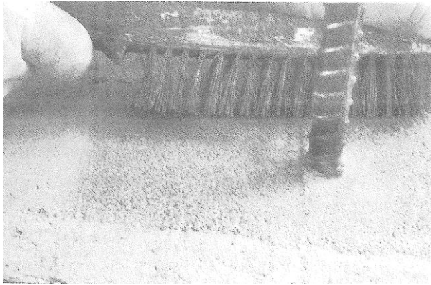
Figure 10: Construction Joint Preparation
