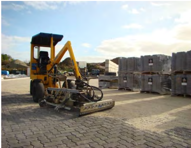
Figure 28: Paver Laying Machine
