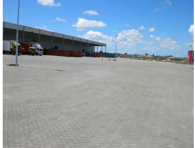
Figure 27: Container and Truck Distribution Warehouses 80 mm Pavers
