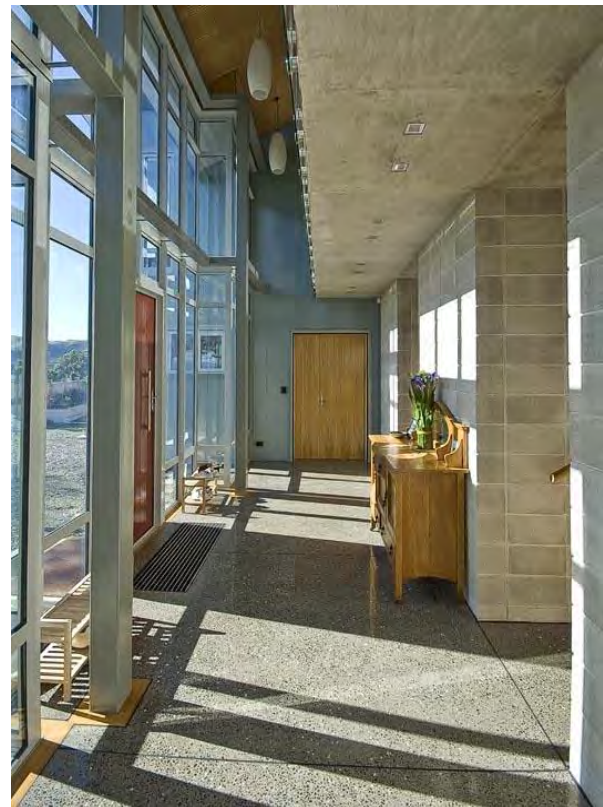
Image: Cranko Architects using principles of passive solar design for a residence in Wellington.
