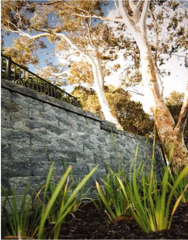
Figure 11: Splitface Finish Retaining Wall
