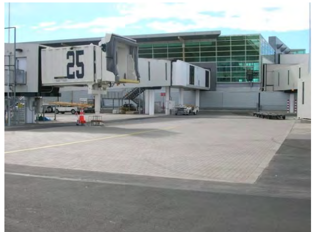
Figure 31: Christchurch Airport Apron Slab 80 mm Pavers
