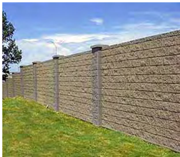
Figure 3: Split Block Wall (Image Source: http://www.blockwall.org/ )
