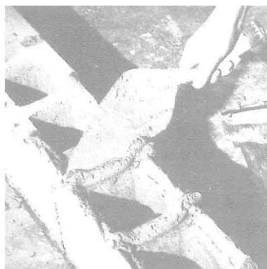
Figure 23 Full mortar bedding
