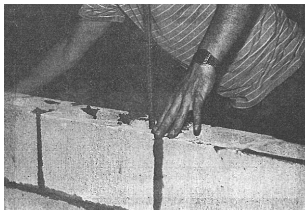
Figure 4: Laying up 15.05 units with reinforcing steel spaced at 800 mm centres
