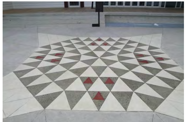
Figure 21: Commercial Flagstone Paving, Wharewaka Building, Wellington
